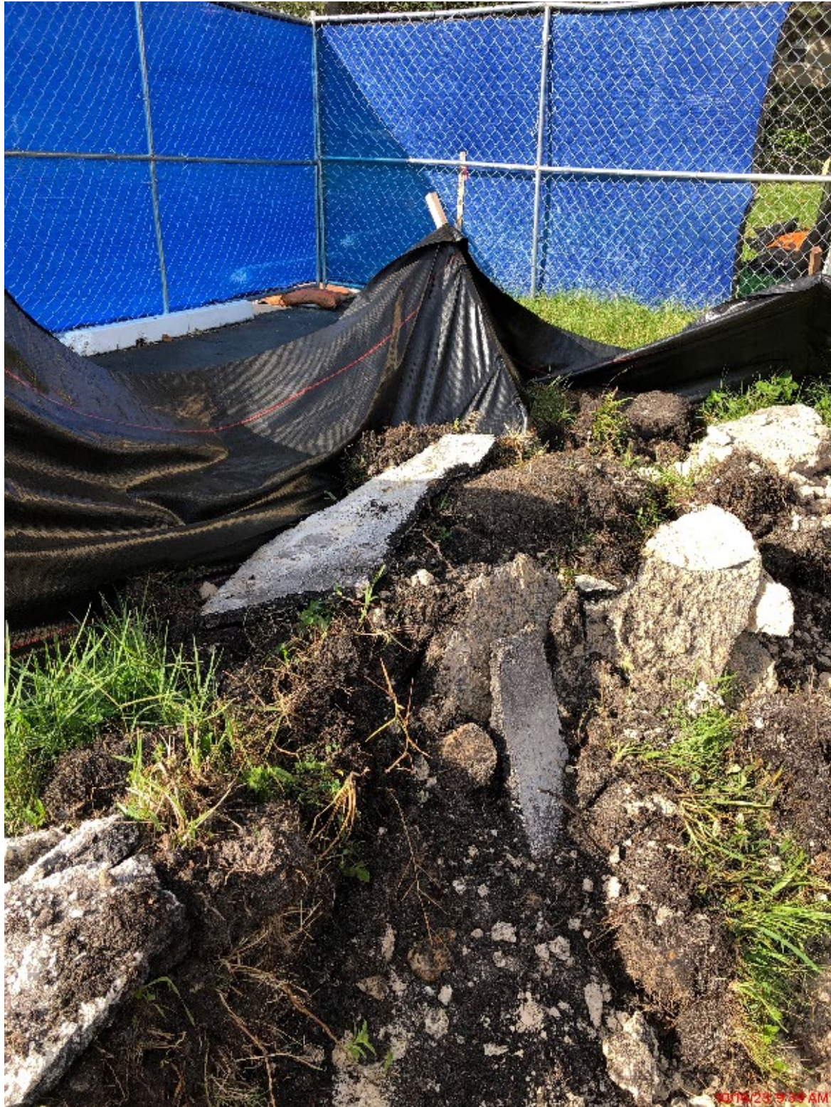
Asphalt Walkway Removed
