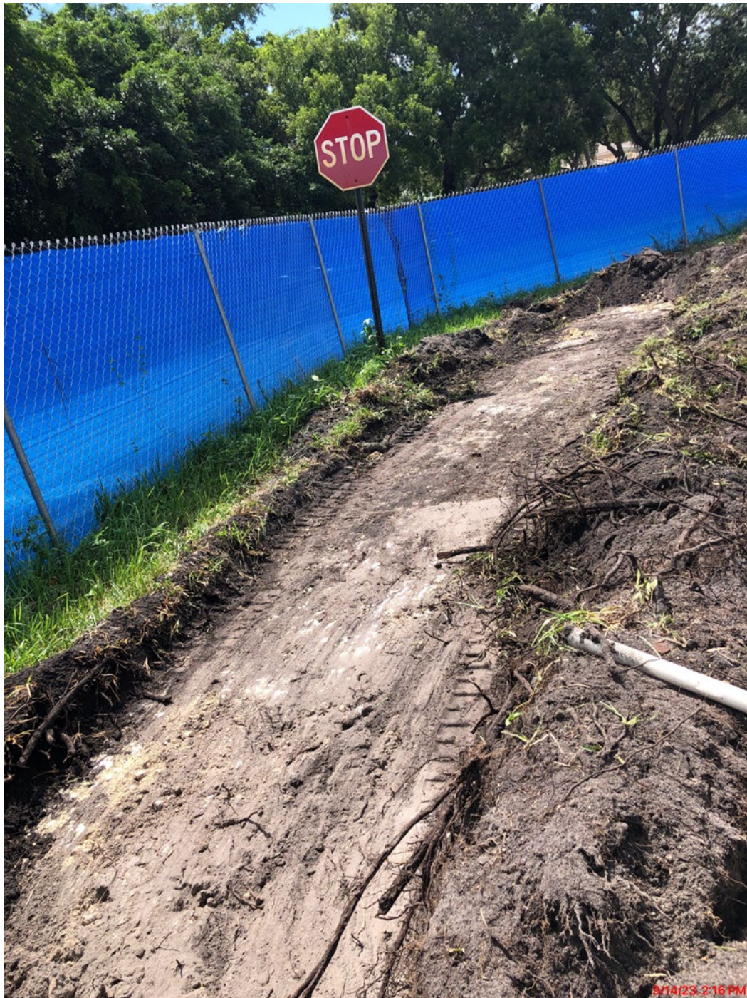
Sidewalk Removal - About 8' wide and 30' long
