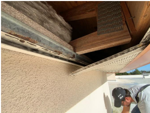
Photo 33 – Main Roof – Tower Walls Overall view of the soffit condition.
