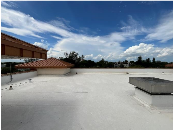
Photo 7 – Main Roof Overall view.
