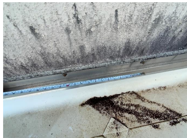
Photo 18 – Main Roof – Interior Tower Walls Overall view of the existing TPO roof counter-flashing fastener measurements.
