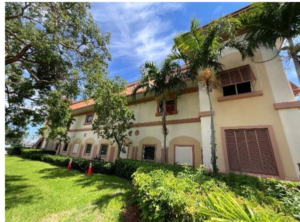
Photo 6 – North Elevation Overall view.
