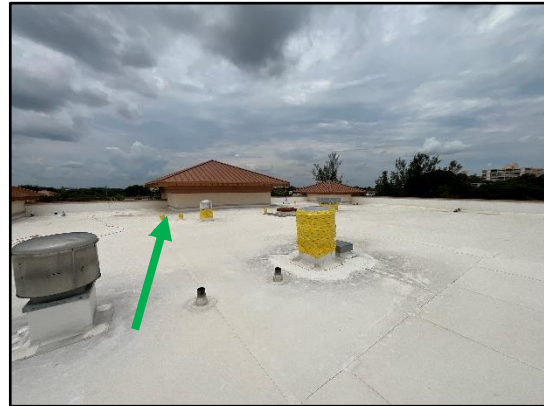
Figure 3 – Overall view of the Main Roof Towers, West Elevation.
