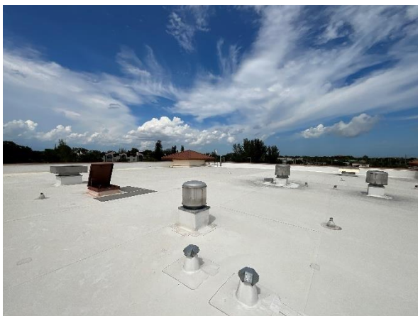
Photo 9 – Main Roof Overall view.
