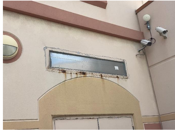
Photo 46 – Main Roof – Tower Walls Overall view of the exterior tilt up walls to be recoated.
