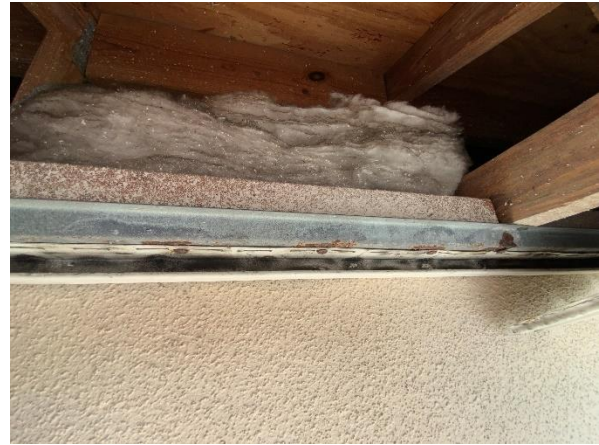
Photo 34 – Main Roof – Tower Walls Overall view of the soffit condition.
