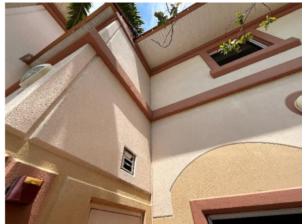
Photo 47 – Exterior Tilt-Up Walls Overall view of the louver perimeter sealant installation.
