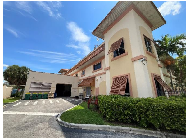
Photo 4 – East Elevation Overall view.
