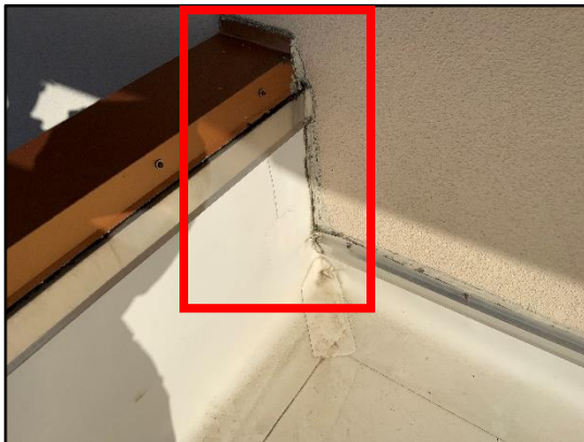
Figure 6 – Overall view of the parapet to conventional stucco transition conditions.
