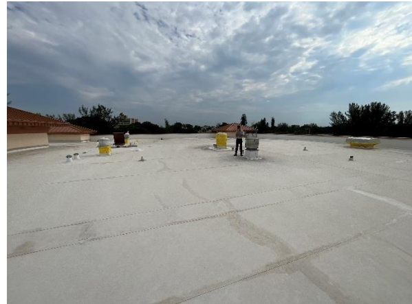
Photo 10 – Main Roof Overall view.
