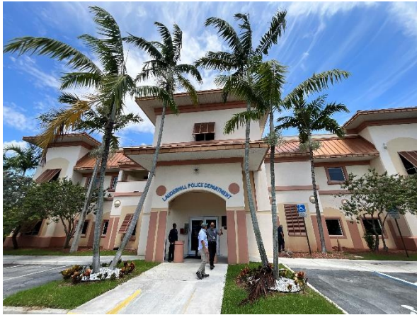
Photo 1 – West Elevation Overall view.
