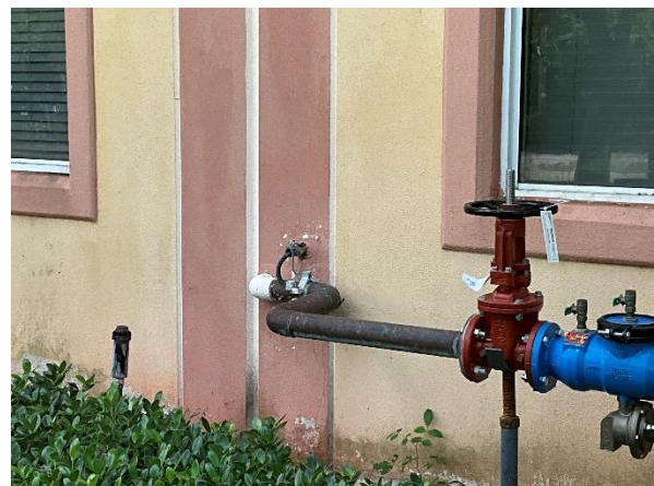
Photo 48 – Exterior Tilt-Up Walls Overall view of the exterior wall pipe penetrations.
