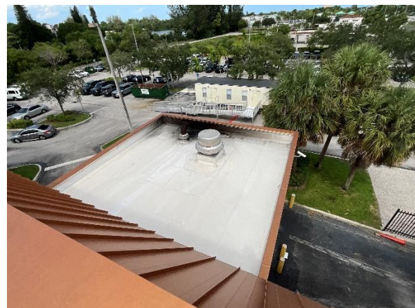
Photo 12 – Lower Roof – East Elevation Overall view.
