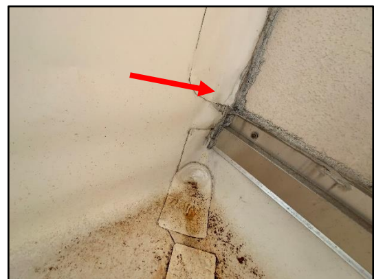
Figure 7 – Overall view of vertical parapet to conventional stucco transition joint.
