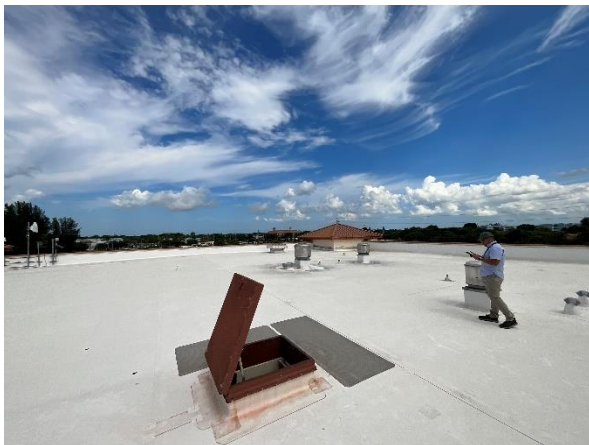
Photo 8 – Main Roof Overall view.
