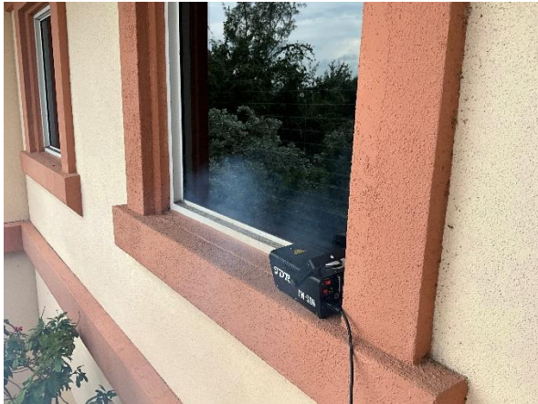
Photo 49 – Exterior Tilt-Up Walls Overall view of the window perimeter sealant installation.
