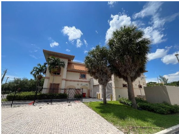
Photo 3 – East Elevation Overall view.
