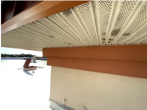
Photo 37 – Main Roof – Tower Walls Overall view of the soffit condition.
