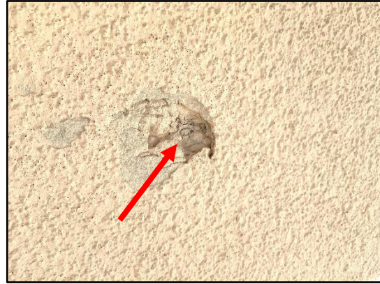
Figure 5 – Overall view of the conventional stucco system and exposed metal lath.
