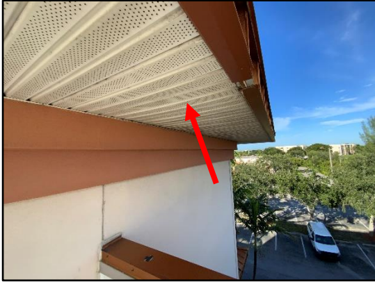
Figure 10 – Overall view of the existing tower soffit vents.
