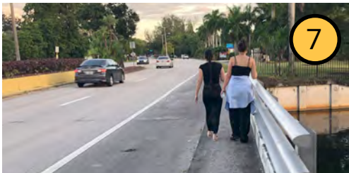
Sidewalk tightens on bridge over Middle River
