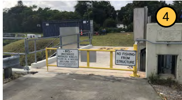
SFWMD Maintenance bridge over the canal
