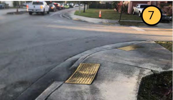
7 Despite the sidewalk curb ramps with detectable warnings, there are no marked crosswalks
