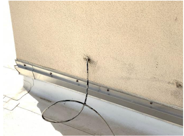
Photo 52 – Main Roof – Tower Walls Overall view of the wire penetrations sealant installation.
