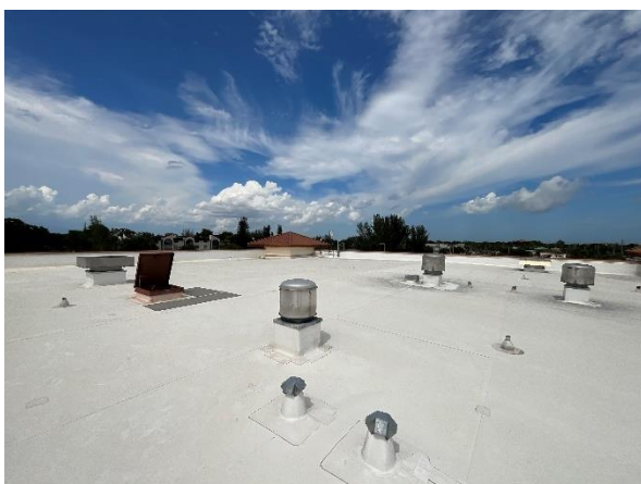
Photo 9 – Main Roof Overall view.
