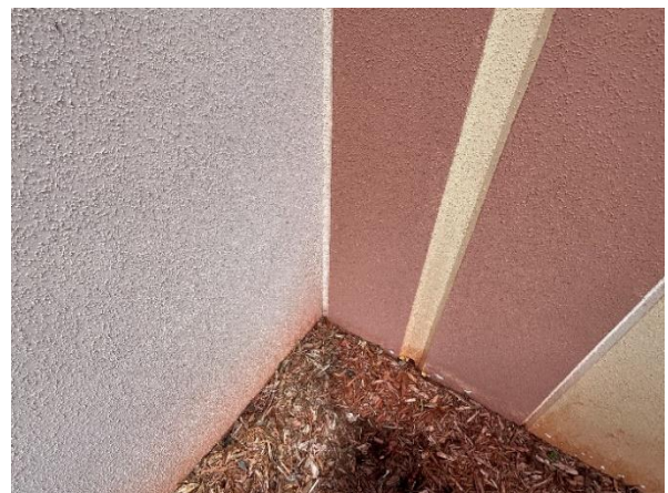
Photo 54 – Exterior Tilt-Up Walls Overall view of an inside corner panel wall joint to be removed and replaced.
