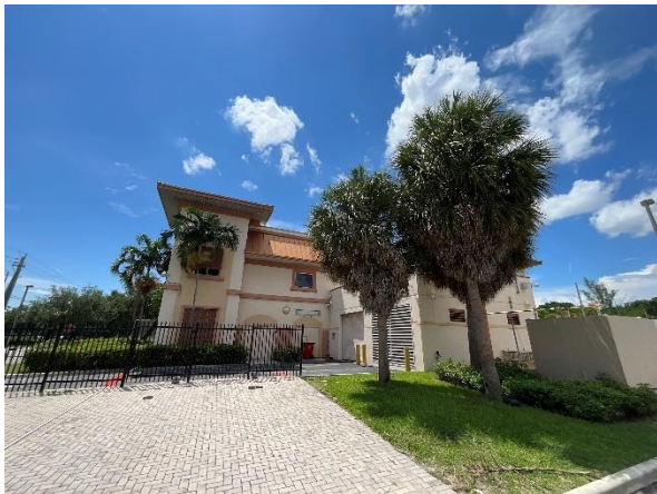
Photo 3 – East Elevation Overall view.
