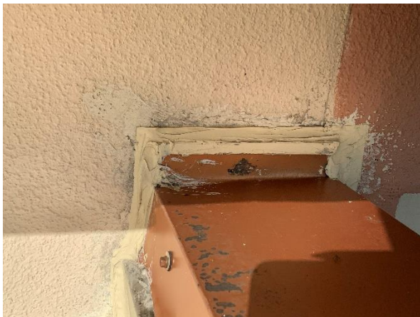
Photo 26 – Main Roof – Interior Tower Walls Overall view of the parapet coping cap to adjacent conventional stucco wall transition.
