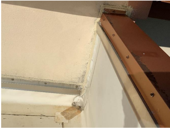
Photo 25 – Main Roof – Interior Tower Walls Overall view of the parapet coping cap to adjacent conventional stucco wall transition.
