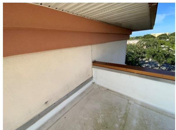
Photo 24 – Main Roof – Interior Tower Walls Overall view of the parapet coping cap to adjacent tilt-up wall transition.
