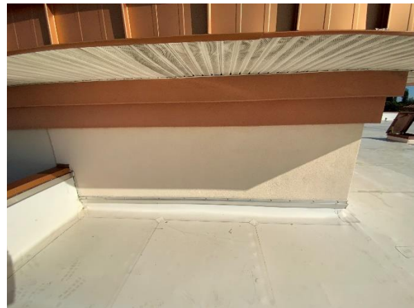
Photo 29 – Main Roof – Tower Walls Overall view of West Center Tower decorative foam trim band.
