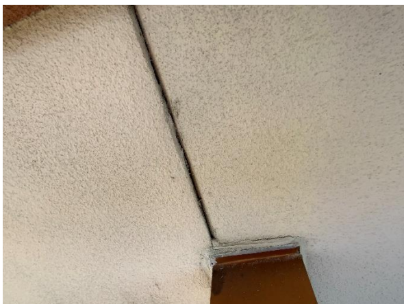
Photo 15 – Main Roof – Interior Tower Walls Overall view of the existing conventional stucco to tilt-up wall transition.
