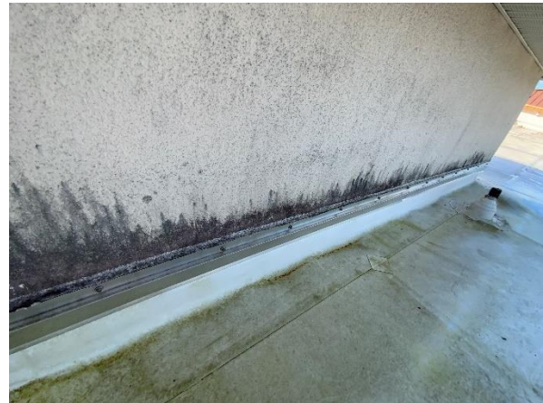
Photo 17 – Main Roof – Interior Tower Walls Overall view of the existing conventional stucco counter-flashing condition.
