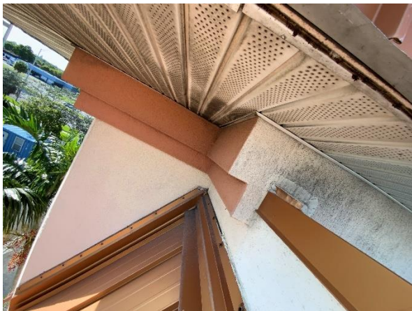
Photo 32 – Main Roof – Tower Walls Overall view of Corner Tower decorative foam trim band.
