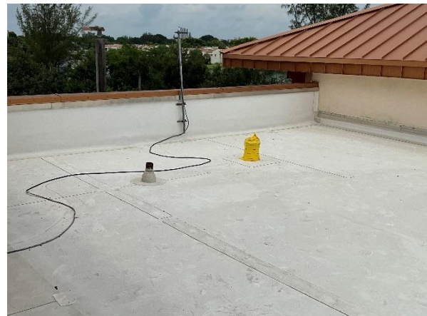
Photo 11 – Main Roof Overall view.
