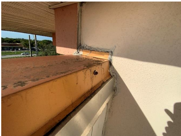
Photo 20 – Main Roof – Interior Tower Walls Overall view of the parapet coping cap to adjacent conventional stucco wall transition.
