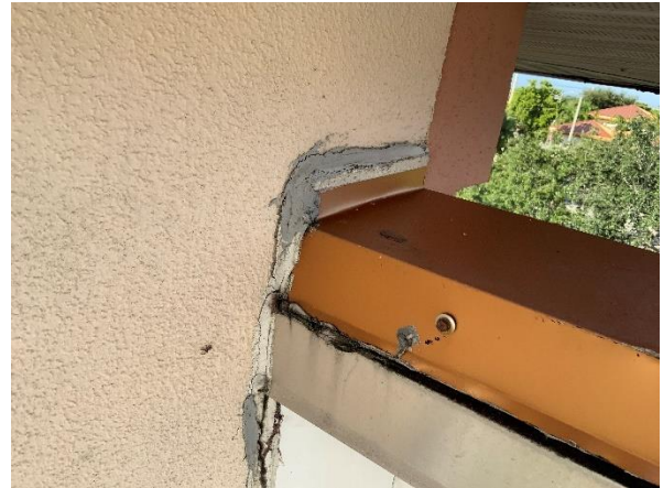
Photo 22 – Main Roof – Interior Tower Walls Overall view of the parapet coping cap to adjacent conventional stucco wall transition.
