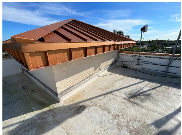
Photo 42 – Main Roof – Tower Walls Overall view of the metal Tower Roof eave fascia condition.
