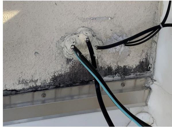
Photo 16 – Main Roof – Interior Tower Walls Overall view of the wire penetrations in the conventional stucco system.
