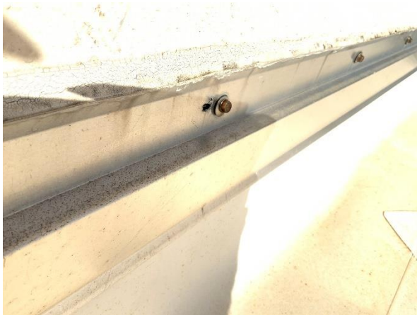
Photo 14 – Main Roof – Interior Tower Walls Overall view of the existing TPO roof counter-flashing condition.
