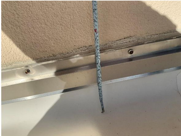
Photo 19 – Main Roof – Interior Tower Walls Overall view of the existing TPO roof counter-flashing measurements.
