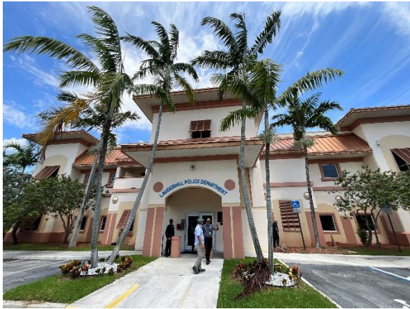
Photo 1 – West Elevation Overall view.
