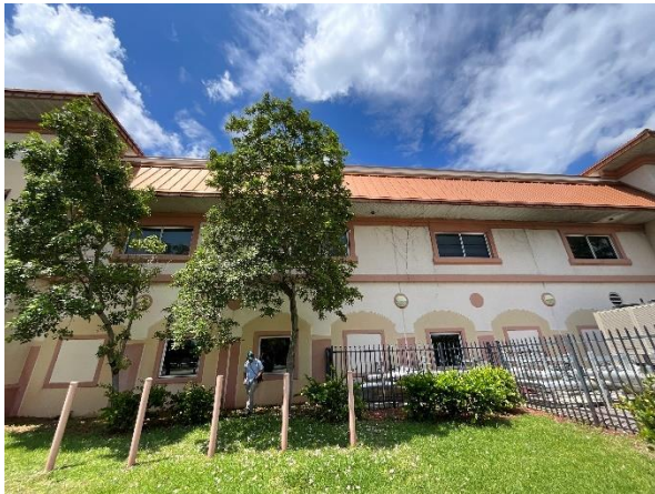
Photo 2 – South Elevation Overall view.
