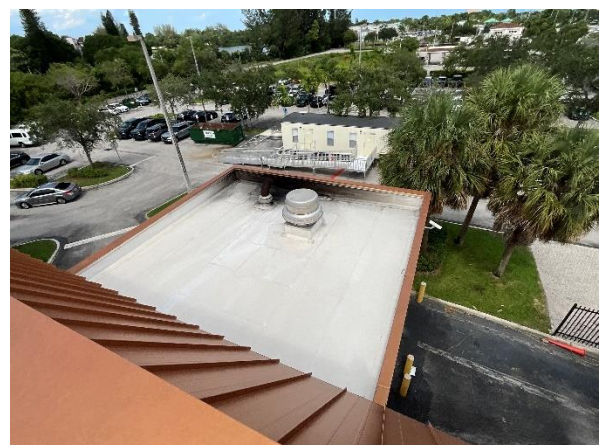
Photo 12 – Lower Roof – East Elevation Overall view.
