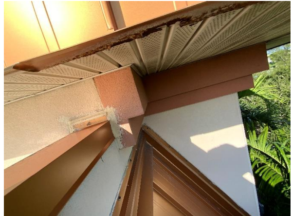
Photo 40 – Main Roof – Tower Walls Overall view of the damaged metal Tower Roof eave fascia condition.
