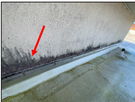
Figure 12 – Overall view of the existing exterior coating condition along the conventional stucco.
