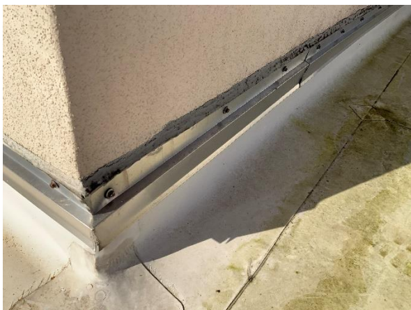
Photo 51 – Main Roof – Tower Walls Overall view of the metal roof counterflashing needing sealant at the TPO interface.
