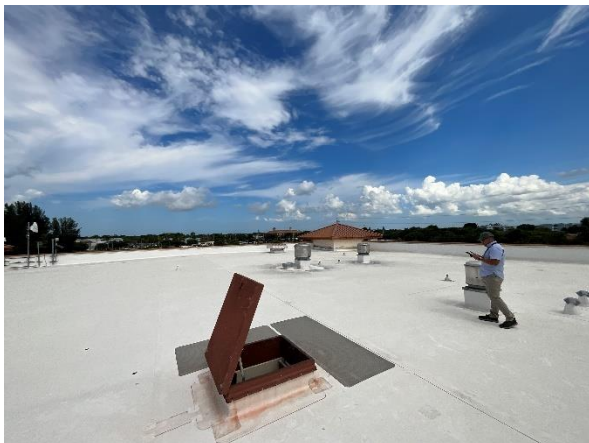
Photo 8 – Main Roof Overall view.
