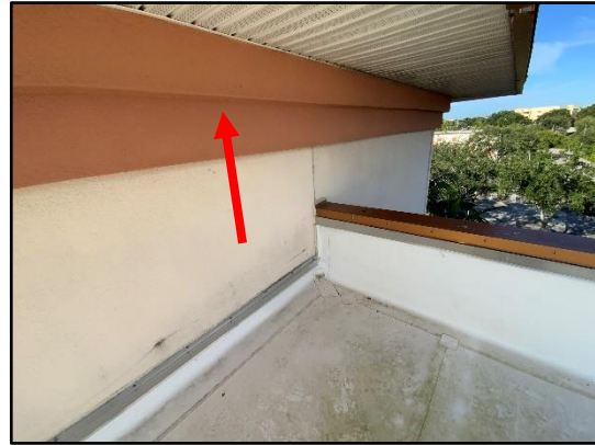
Figure 9 – Overall view of the existing foam trim bands along the Center West Tower.
