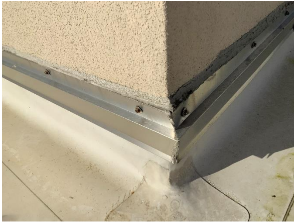
Photo 13 – Main Roof – Interior Tower Walls Overall view of the existing conventional stucco counter-flashing condition.
