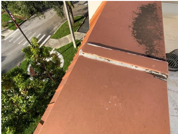
Photo 50 – Main Roof – Parapet Walls Overall view of the coping cap splice cover sealant installation.
