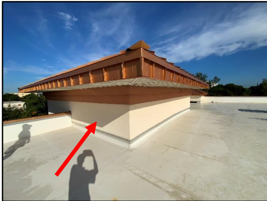
Figure 4 – Overall view of the conventional stucco on the Roof Tower interior walls.
