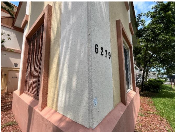
Photo 56 – Exterior Tilt-Up Walls Overall view of an outside corner panel wall joint to be removed and replaced.
