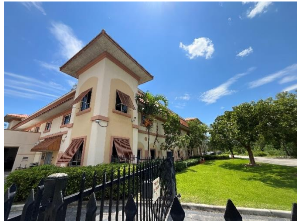
Photo 5 – North Elevation Overall view.
