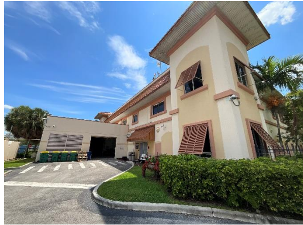
Photo 4 – East Elevation Overall view.
