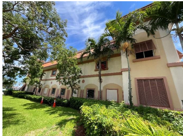
Photo 6 – North Elevation Overall view.
