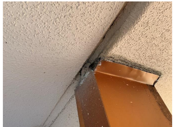
Photo 23 – Main Roof – Interior Tower Walls Overall view of the parapet coping cap to adjacent tilt-up wall transition.
