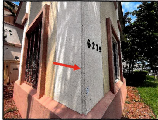
Figure 17 – Overall view of an outside corner panel wall joint to be removed and replaced.
