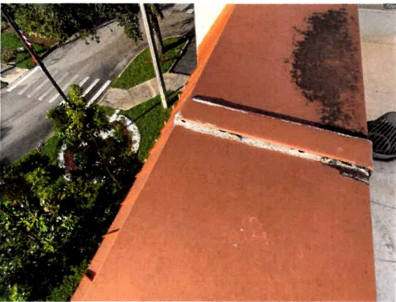
Photo 50 – Main Roof – Parapet Walls Overall view of the coping cap splice cover sealant installation.
