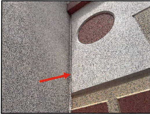
Figure 16 – Overall view of an inside corner panel wall joint to be removed and replaced.
