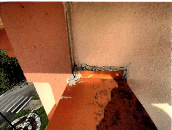
Photo 21 – Main Roof – Interior Tower Walls Overall view of the parapet coping cap to adjacent conventional stucco wall transition.
