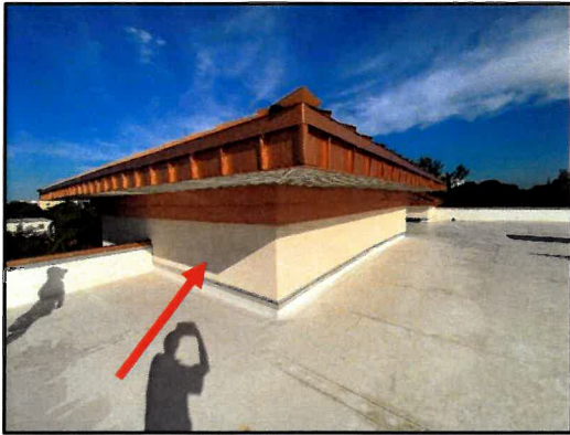
Figure 4 – Overall view of the conventional stucco on the Roof Tower interior walls.
