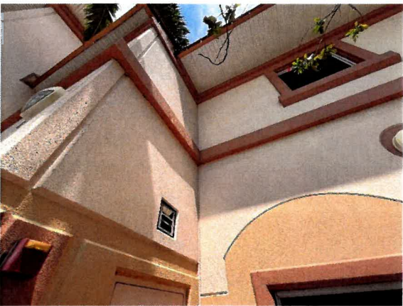
Photo 44 – Exterior Tilt-Up Walls Overall view of the exterior tilt up walls to be recoated.
