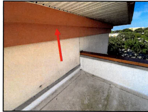
Figure 9 – Overall view of the existing foam trim bands along the Center West Tower.
