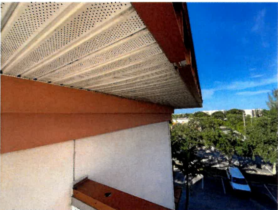
Photo 38 – Main Roof – Tower Walls Overall view of the damaged metal Tower Roof eave fascia condition.
