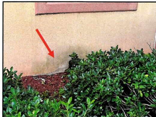
Figure 13 – Overall view of the existing exterior coating condition along the tilt-up panel walls.
