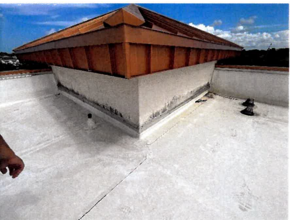
Photo 45 – Main Roof – Tower Walls Overall view of the exterior framed Tower walls to be recoated.
