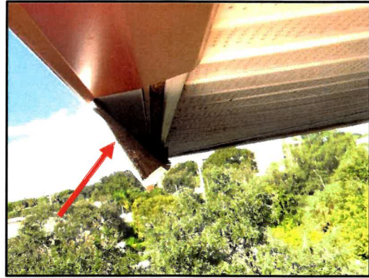
Figure 11 – Overall view of damaged roof fascia.
