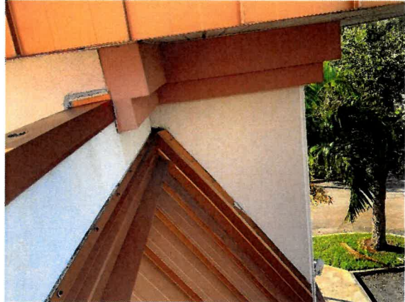
Photo 28 – Main Roof – Tower Walls Overall view of Corner Tower decorative foam trim band.
