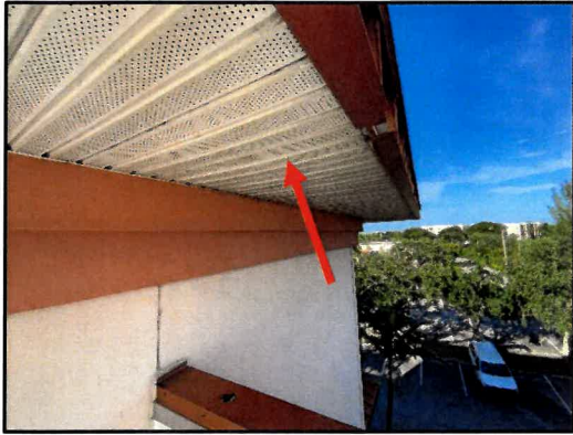
Figure 10 – Overall view of the existing tower soffit vents.
