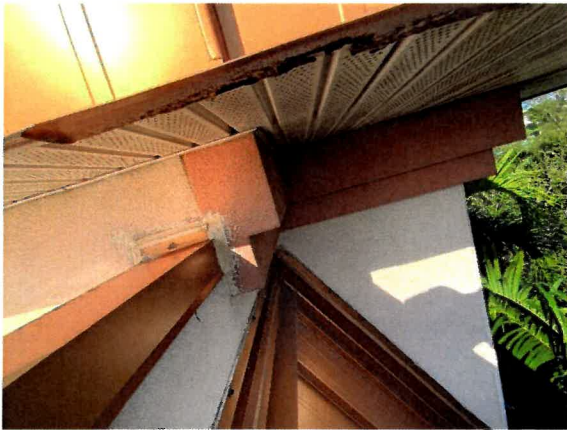
Photo 31 – Main Roof – Tower Walls Overall view of Corner Tower decorative foam trim band.
