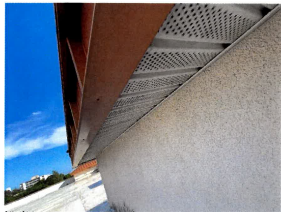
Photo 53 – Main Roof – Tower Walls Overall view of the soffit vent sealant installation interface.
